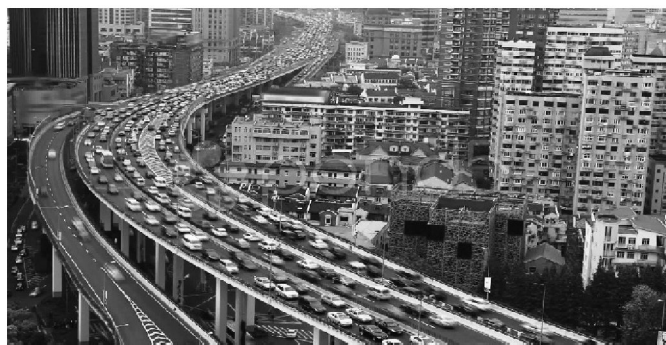
Figure 1. Dense traffic as accident risk on flyovers
