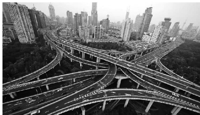
Figure 3. Possible accident risk at sharp bend on bridges [1]
