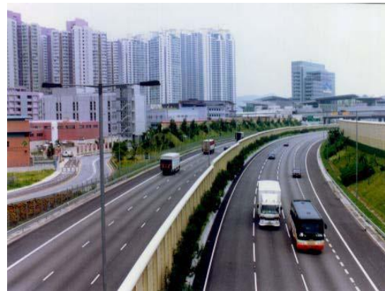
Figure 13: Vegetated Barrier
