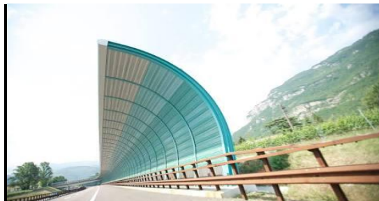
Figure 11: Curved Barrier
