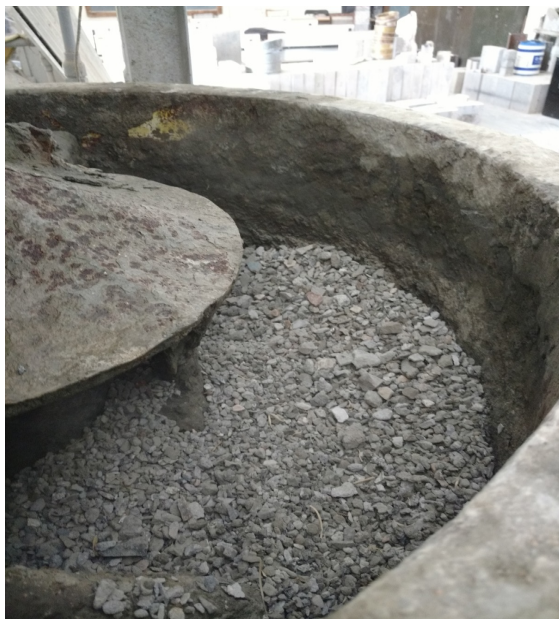
Figure 2: Figure of dry mixing of materials
