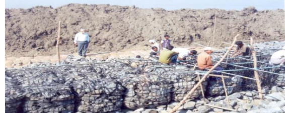
Figure 8: Gabions filled with sandbags [23]
