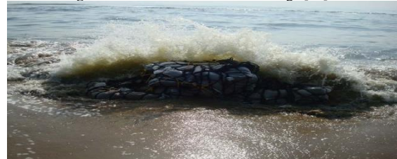
Figure 9: Gabions filled with sandbags at Ocean [23]
