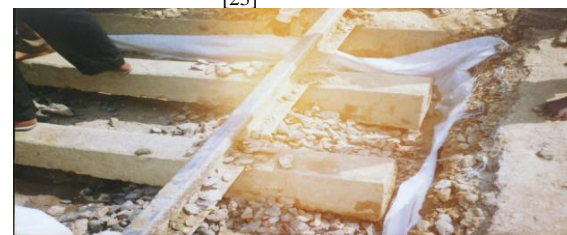
Figure 2: Geotextile layer applied below railway track [23]
